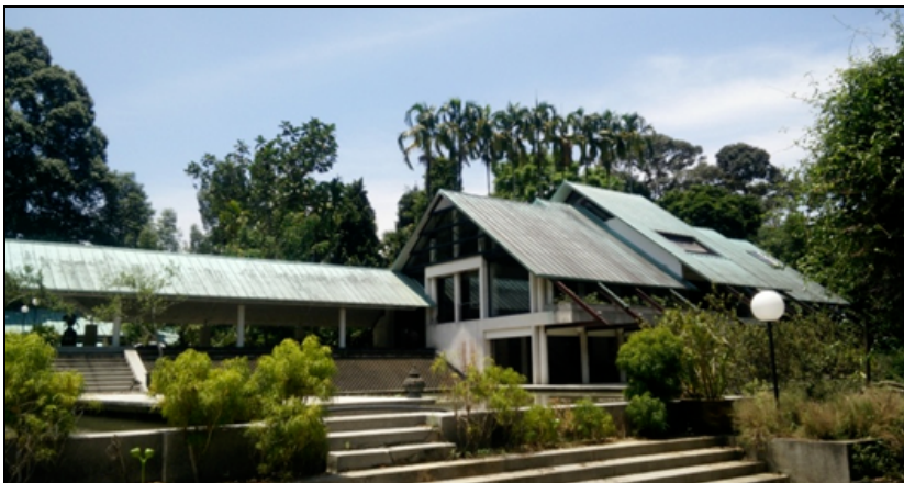
Figure 5. The roof design dominates the physical appearance of the house. It has the same roof language with the covered loggia. The roof of the main house is based on the Malay traditional home
