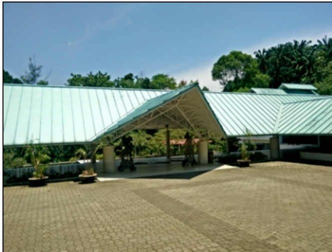
Figure 4. The covered loggia at the same time created the visual parameter for the internal area of the main house which is located at the back of the covered loggia
